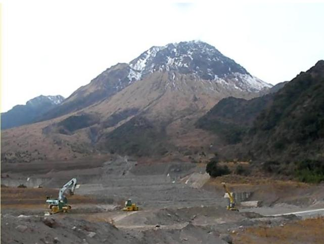
**Fig. 4.** Unmanned construction system at Fugen-dake of Mount Unzen
